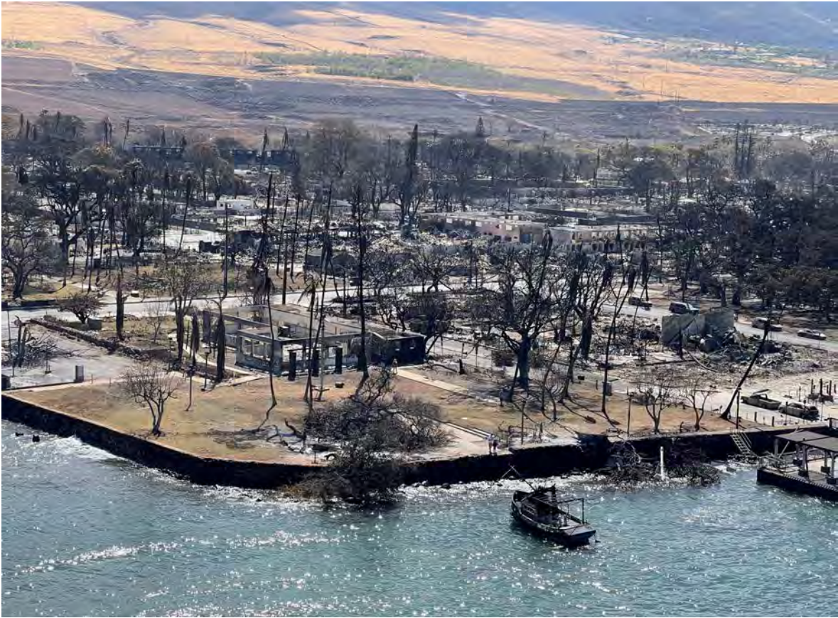
Figure 7: Lahaina, post-fire. (August 11, 2023; Hawai'i Department of Land and Natural Resources.)
