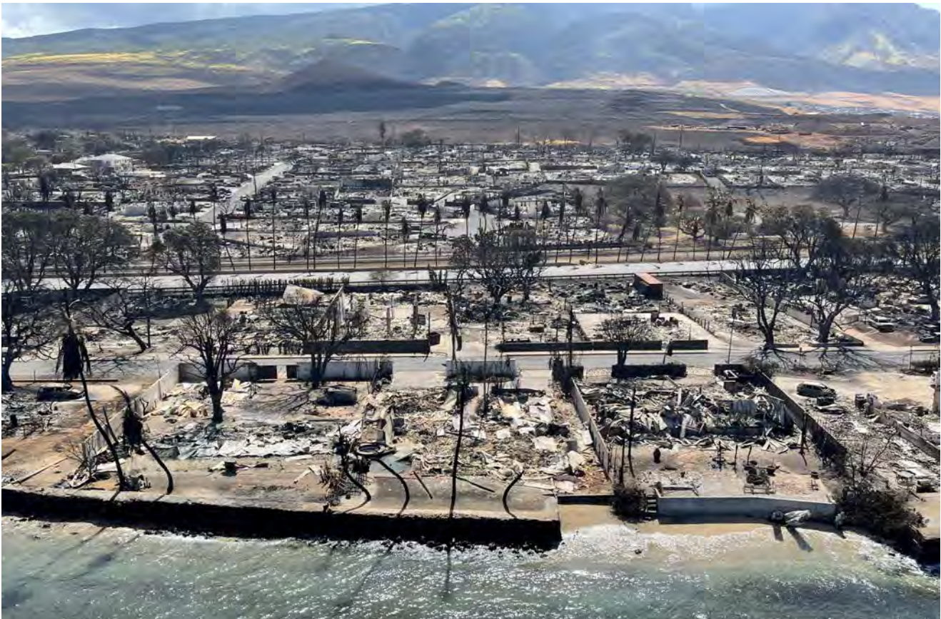
Figure 1: Lahaina, post-fire. (August 11, 2023; Hawai‘i Department of Land and Natural Resources.)
